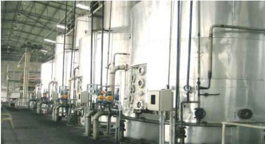
BATCH PANS WITH MECHANICAL CIRCULATOR
