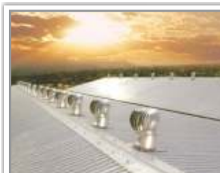
Rooftop Wind Ventilator
